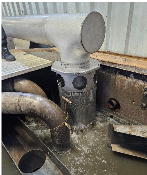
Photo 8 Outlet strainer for filtering water released into the channel.
