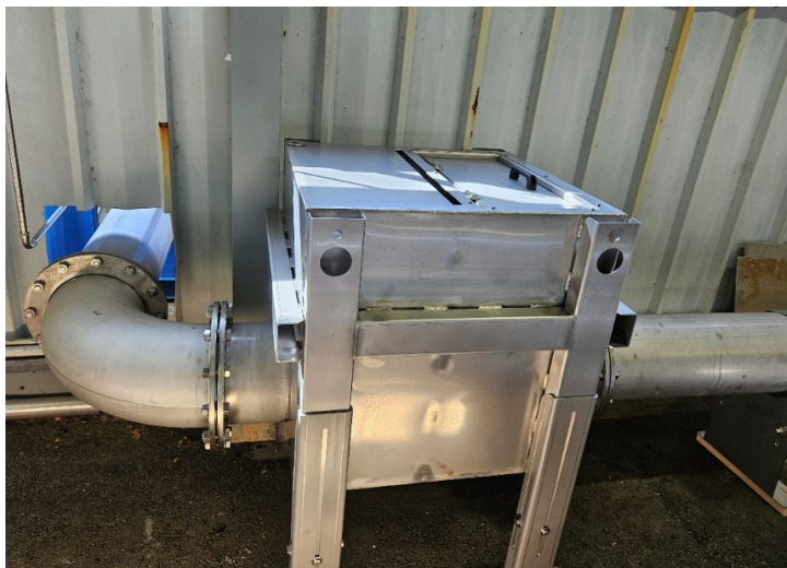
Photo 6 Outlet box with the possibility of adjusting the liquid level after the screen.
